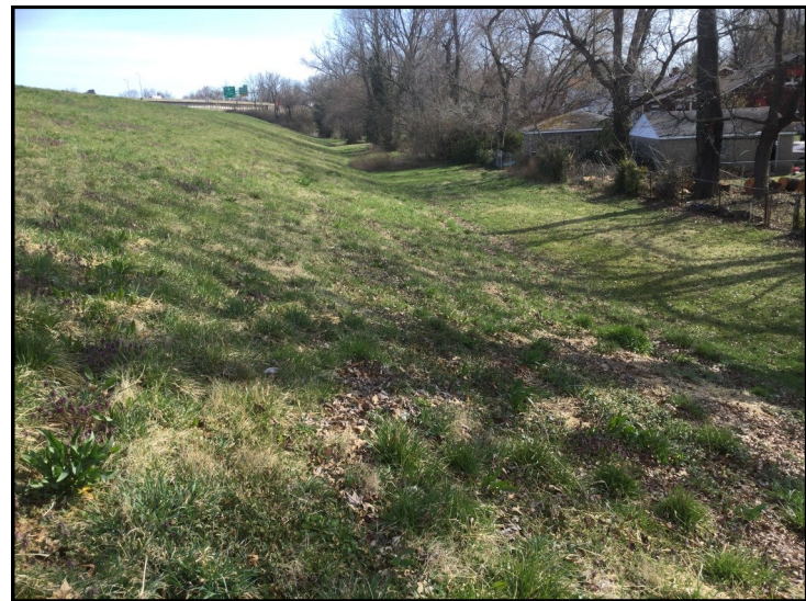
12. View of eastern side of levee, looking northeast.
