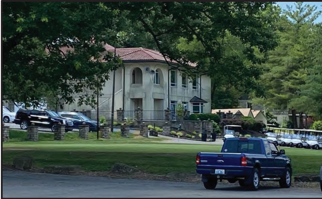
Photo 1. Photo of the rear elevation of the Shawnee Golf Course's Club House facing southwest
