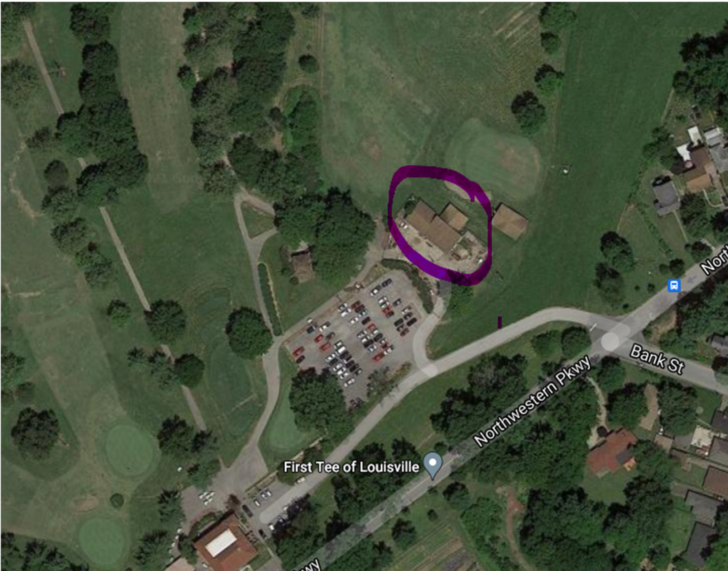
Access along the top of the levee to below the bridge.
