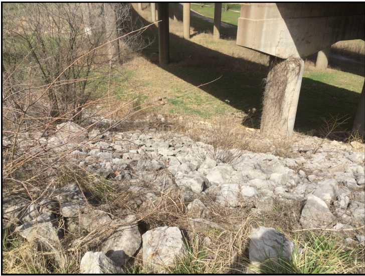
29. View of western side of levee near northern PSL, looking northwest.
