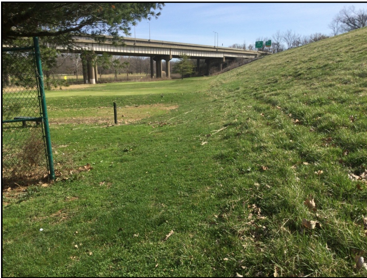
23. View of western side of levee, looking northeast.
