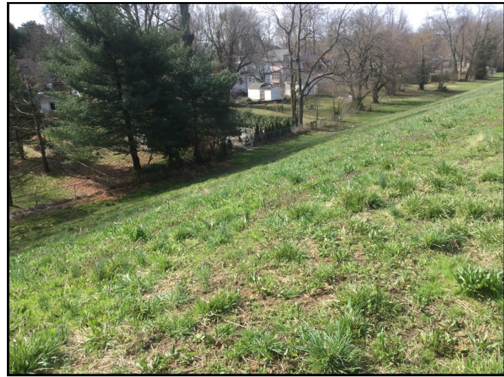
26. View of eastern side of levee from northern PSL, looking south.
