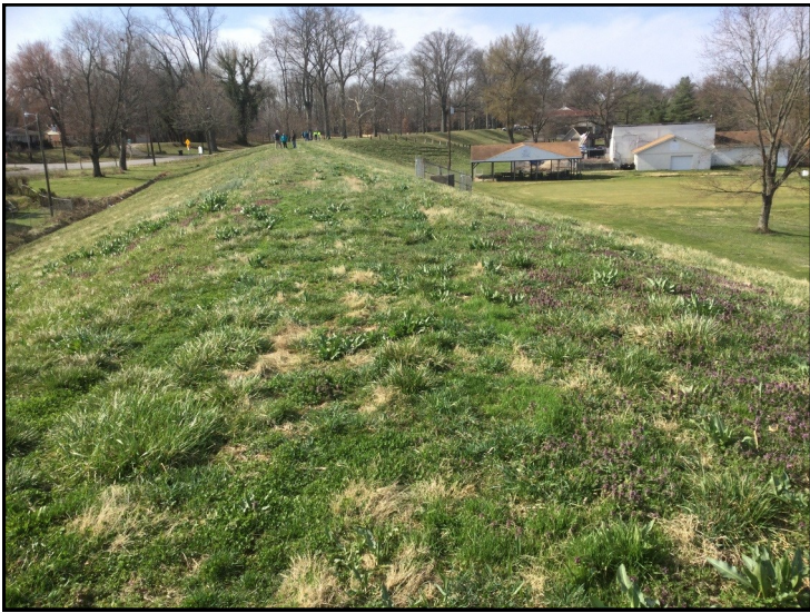
13. View of levee, looking southwest.
