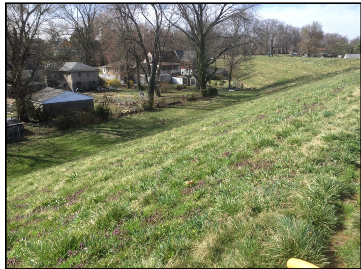
20. View of eastern side of levee, looking southwest.
