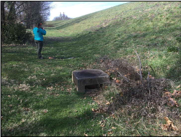
25. View of CV-2 and western side of levee, looking southwest.
