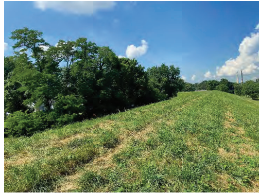
2. View on top of levee facing southwest
