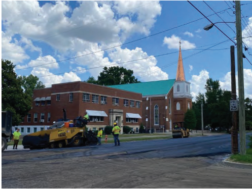
13. Good Shepherd Church on the north side of Rudd Avenue facing northeast from N 36 th Street
