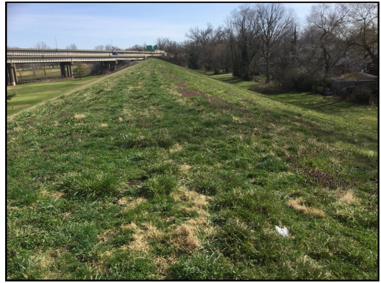
14. View of levee, looking northeast.
