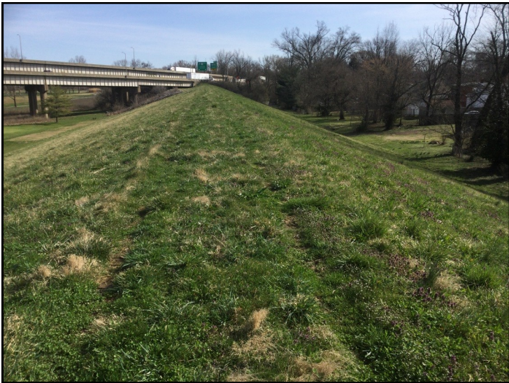
19. View of levee, looking northeast.
