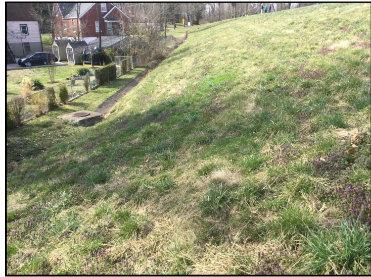
10. View of eastern side of levee, CV 1, and RSD 1, looking southwest.
