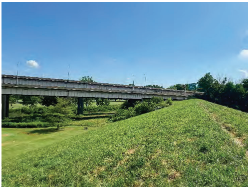
3. View on top of levee facing northeast toward approach bridges
