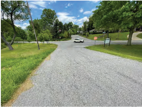
1. View of Shawnee Golf Course entrance facing southeast toward Northwestern Parkway
