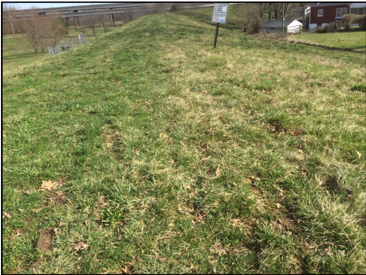
3. View of levee from southern PSL, looking northeast.
