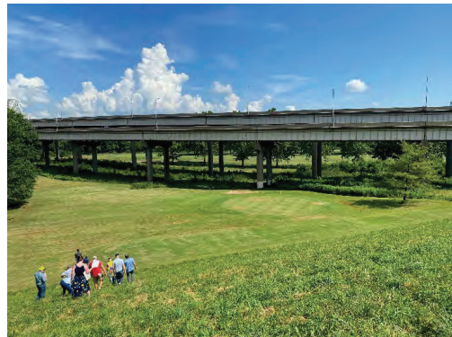
4. View from top of levee north toward approach bridges
