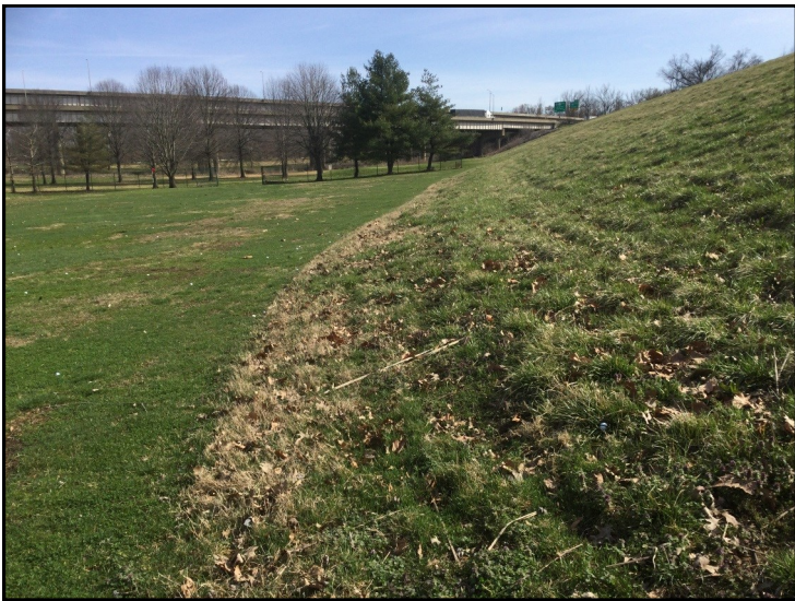
17. View of western side of levee, looking northeast.
