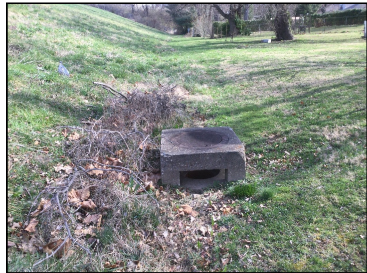
24. View of CV-2 and western side of levee, looking northeast.
