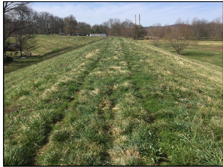
18. View of levee, looking southwest.
