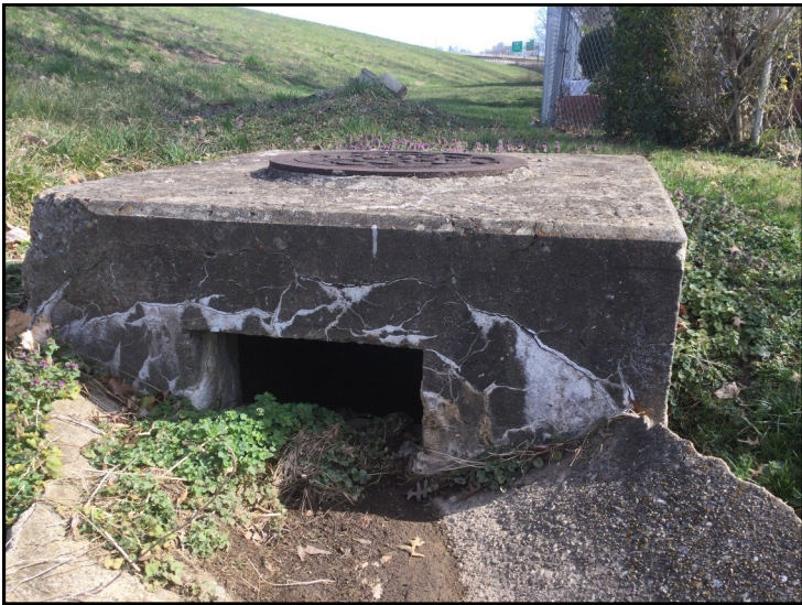
9. View of CV-1 inlet, looking northeast.
