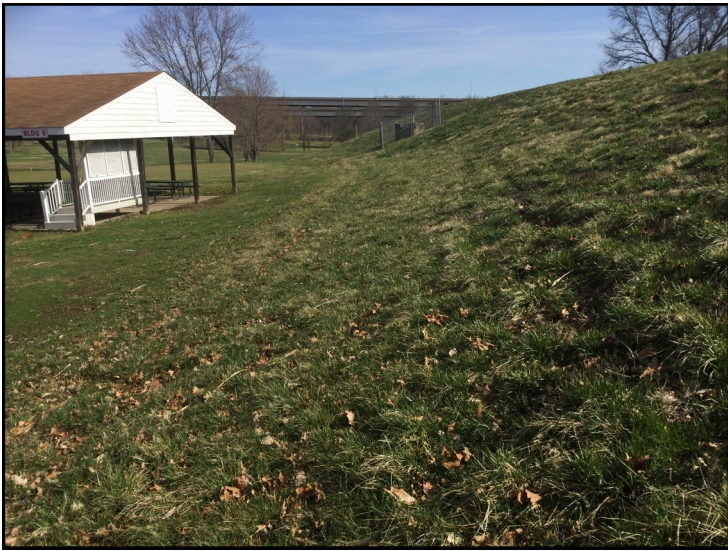
5. View of western side of levee, looking northeast.
