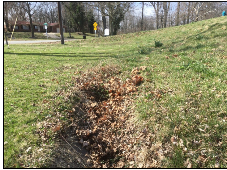
6. View of southern terminal point of Roadside Ditch (RSD) 1, looking southwest.
