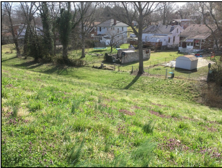
21. View of eastern side of levee, looking east.
