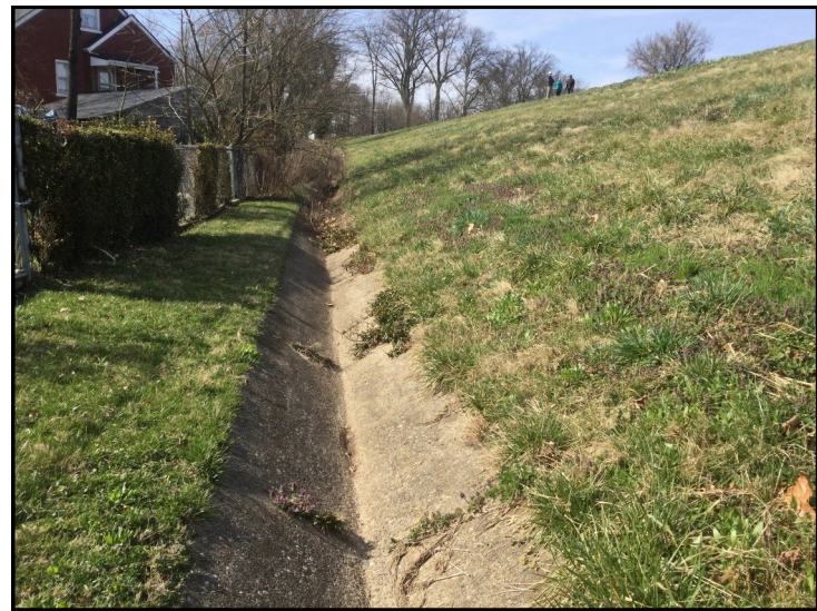
8. View of RSD 1 from Culvert (CV) 1, looking southwest.
