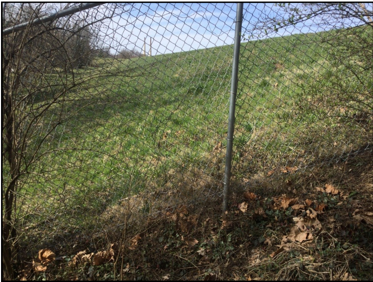
31. View of eastern side of levee from northwestern PSL, looking southwest.
