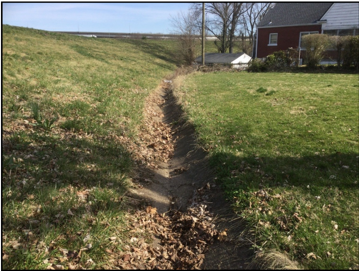
7. View of RSD 1 from its southern terminal point, looking northeast.
